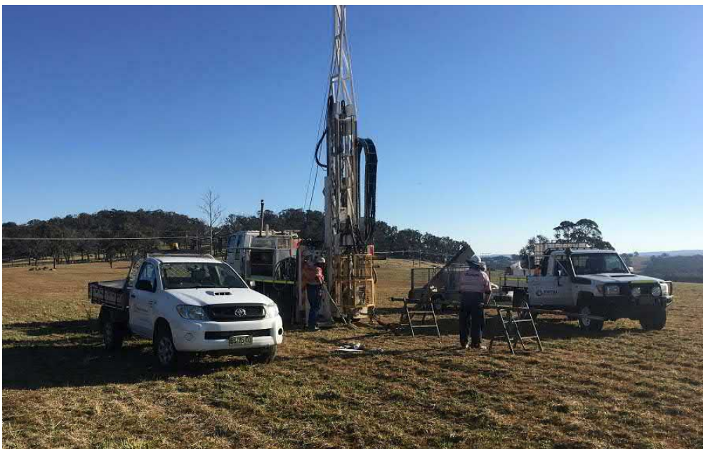
Fig. 3: Typical setup for a geotechnical investigation
